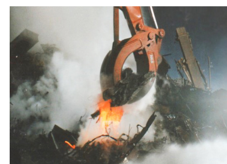
An excavating machine lifts debris dripping with molten metal
